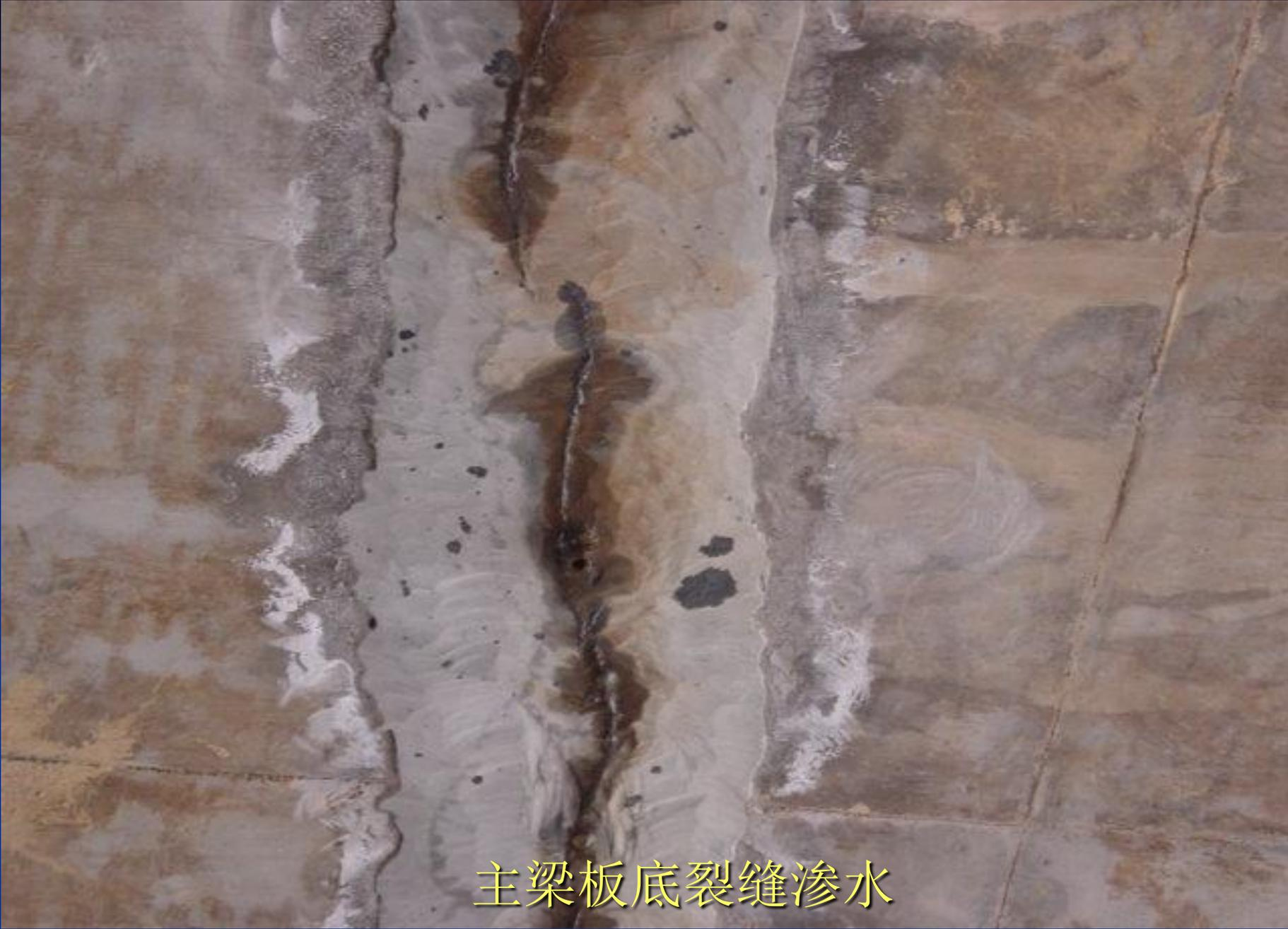
A close-up photograph of a concrete crack in a main beam slab. The crack is a vertical, irregular fissure running through the center of the frame. The concrete surface is heavily stained with brown and greyish water marks, particularly around the crack. The texture of the concrete is rough and uneven. The lighting is somewhat dim, highlighting the depth of the crack and the surrounding moisture.
